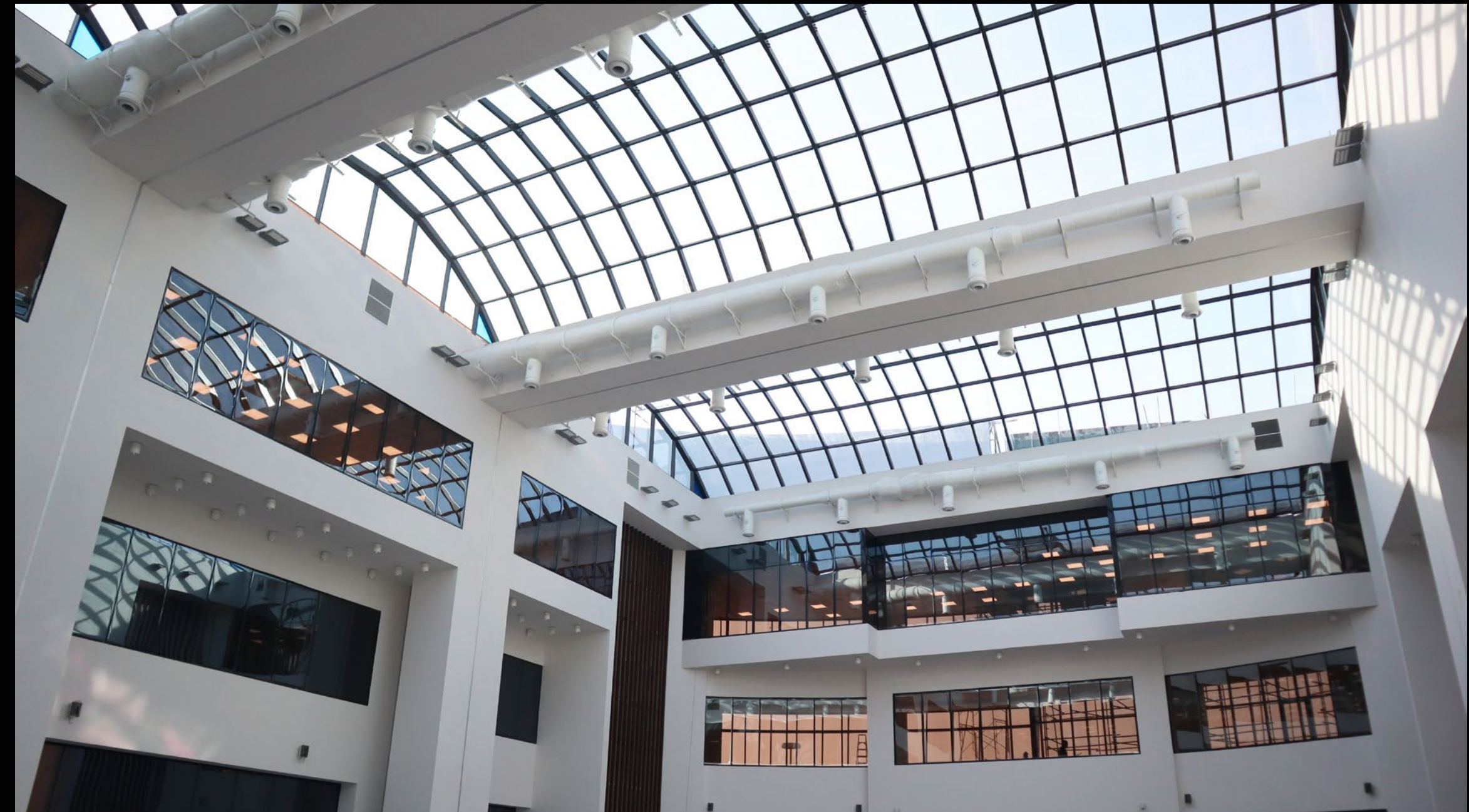
skylight in ministry of sport
